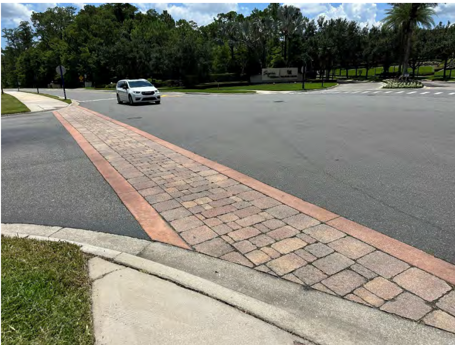
PHOTO 54 ADA ramp/Sidewalk- broken/cracking
