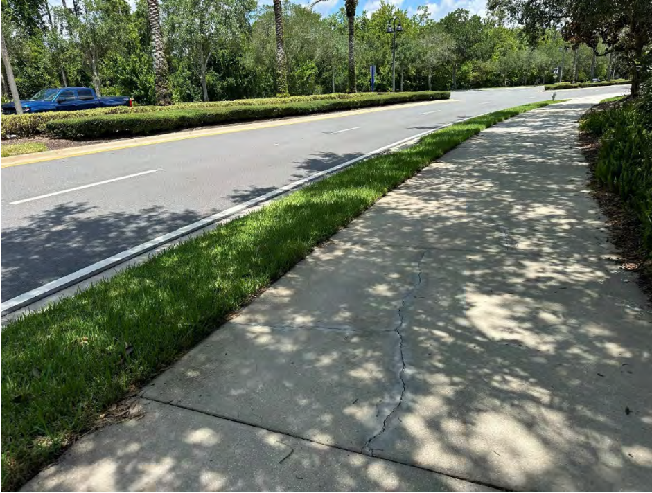
PHOTO 45 Sidewalk- broken/cracking
