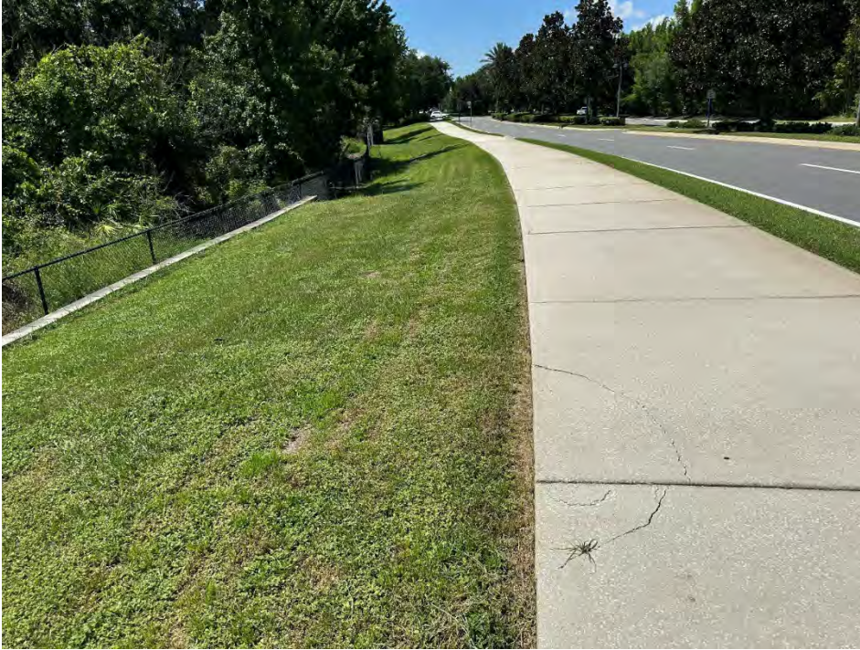
PHOTO 33 Sidewalk- broken/cracking
