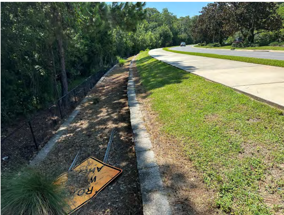
PHOTO 24 Old MOT signage- left behind
