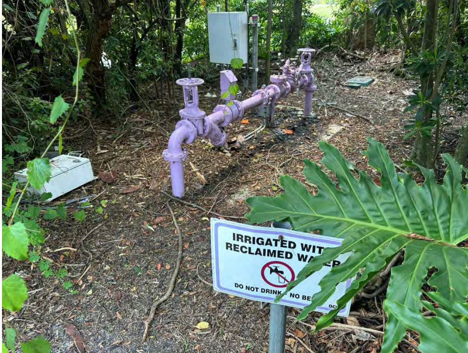
PHOTO 65 Old electrical panel- left behind
