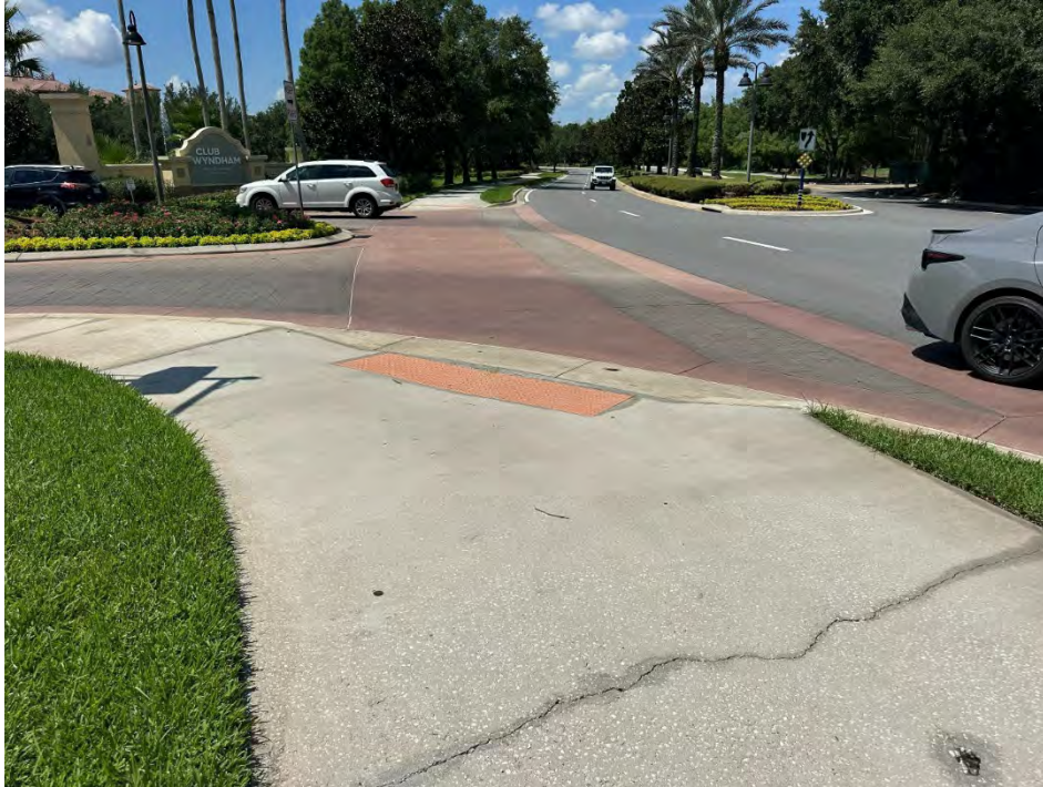
PHOTO 37 Sidewalk- broken/cracking
