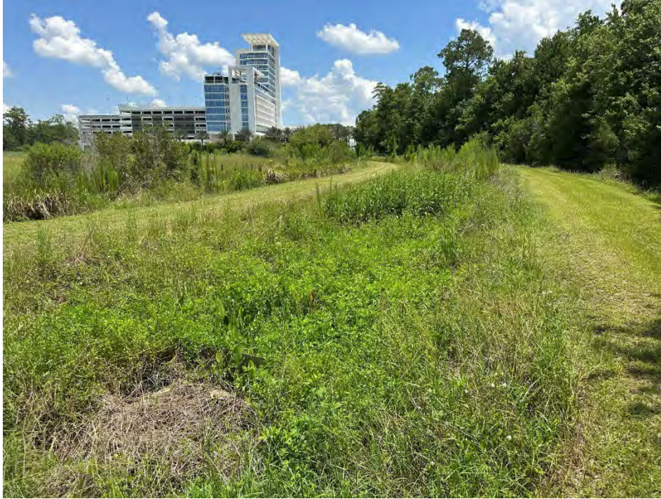
PHOTO 77 Control structure- excess vegetation growth
