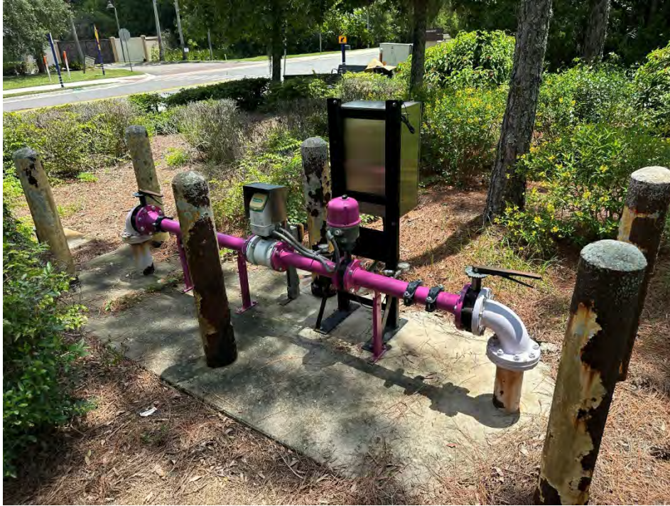
PHOTO 59 Bollards- rusted
