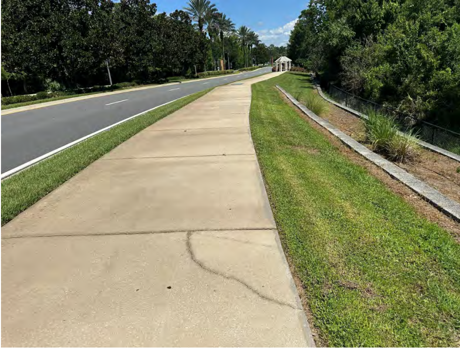
PHOTO 23 Sidewalk- broken/cracking
