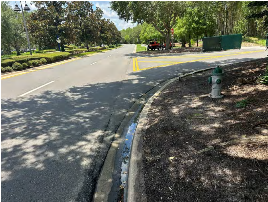
PHOTO 70 Pavement- minor birdbath
