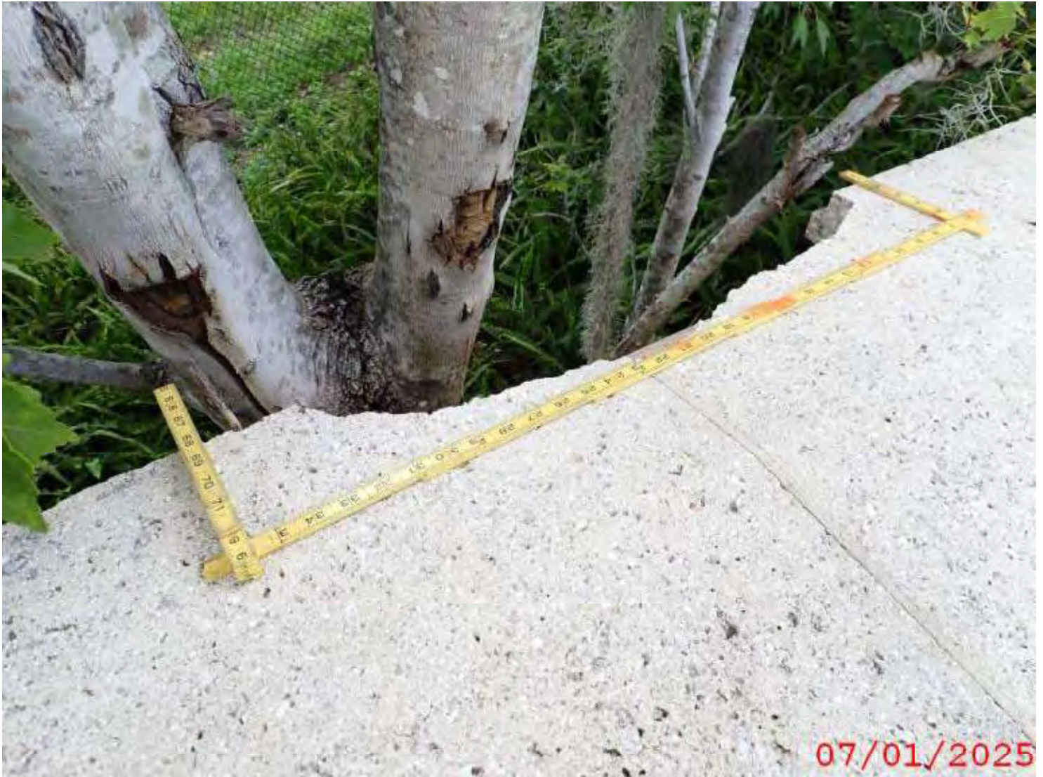
Photo 4: Element 331 Re Conc Bridge Railing
