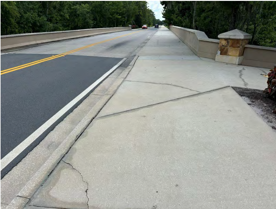
PHOTO 80 Sidewalk- broken/cracking
