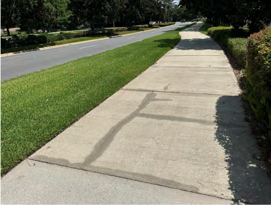
PHOTO 39 Sidewalk- broken/cracking
