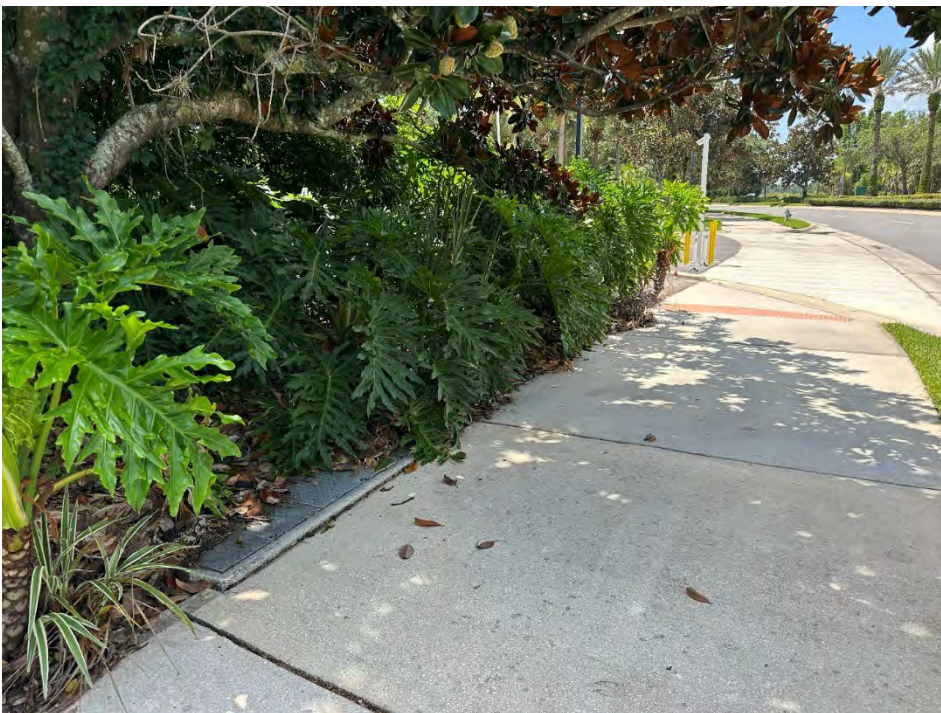
PHOTO 40 Electrical junction box- excess debris covering
