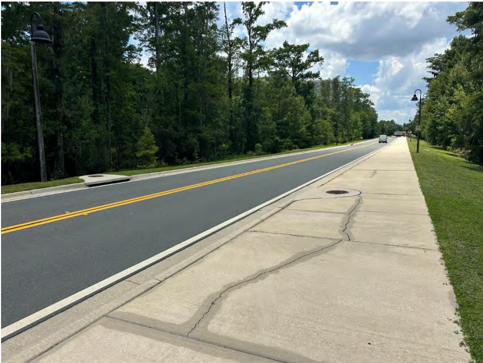
PHOTO 72 Sidewalk- broken/cracking
