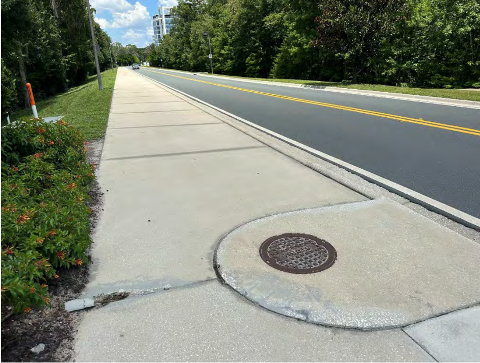
PHOTO 79 Sidewalk- broken/cracking
