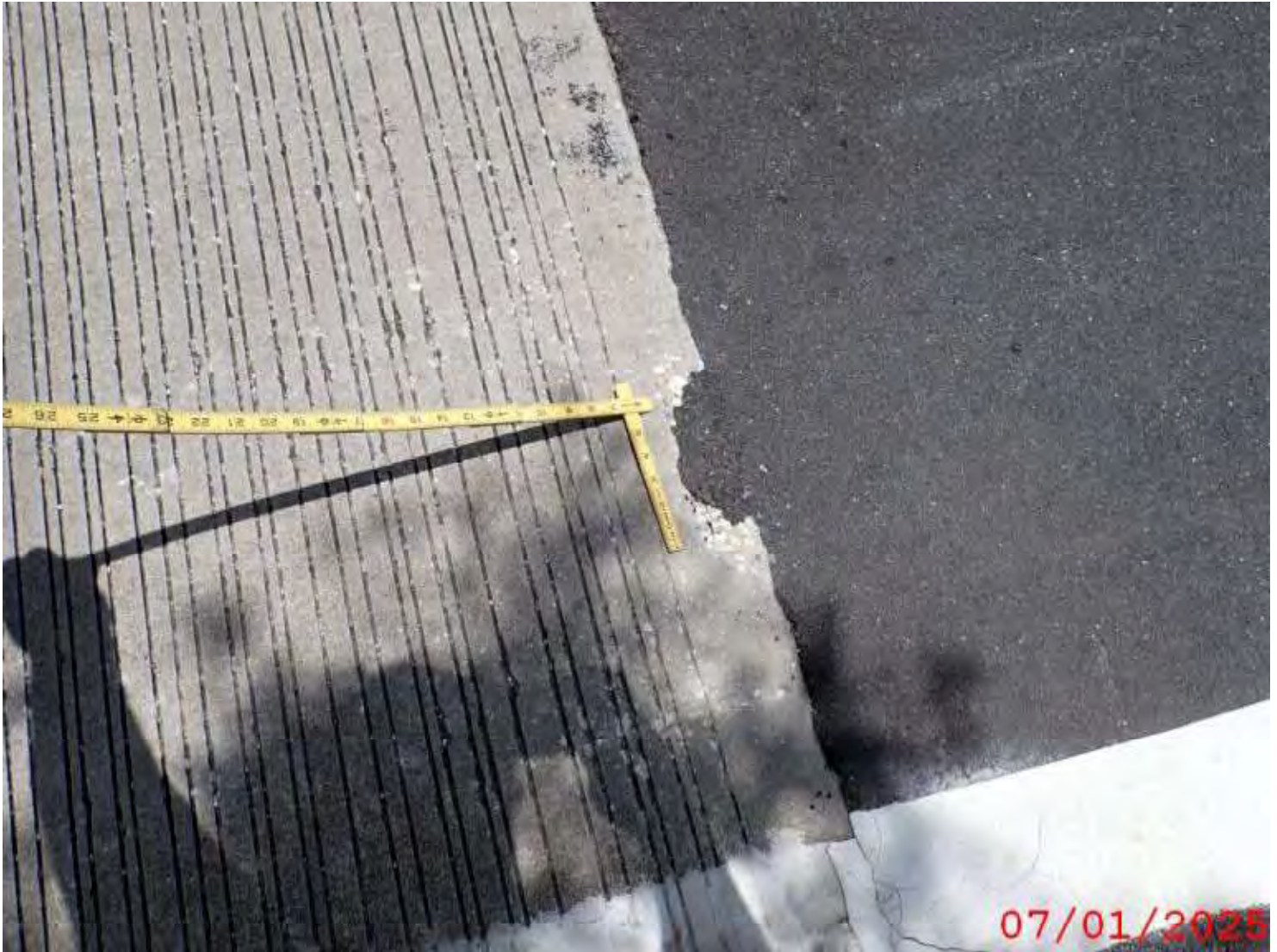
Photo 2: Element 321 Re Conc Approach Slab
