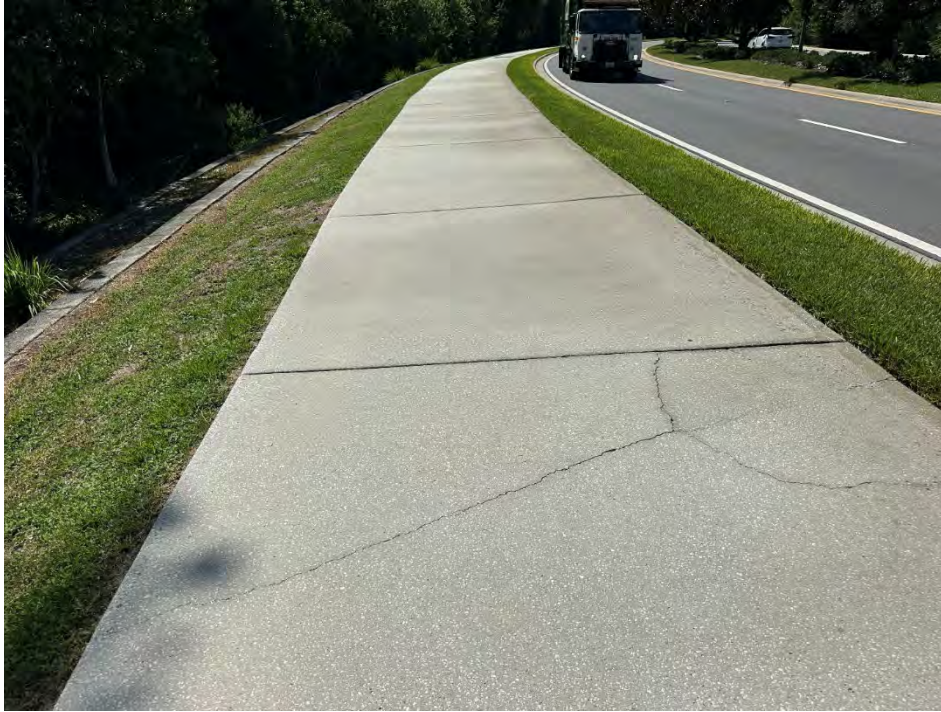
PHOTO 25 Sidewalk- broken/cracking
