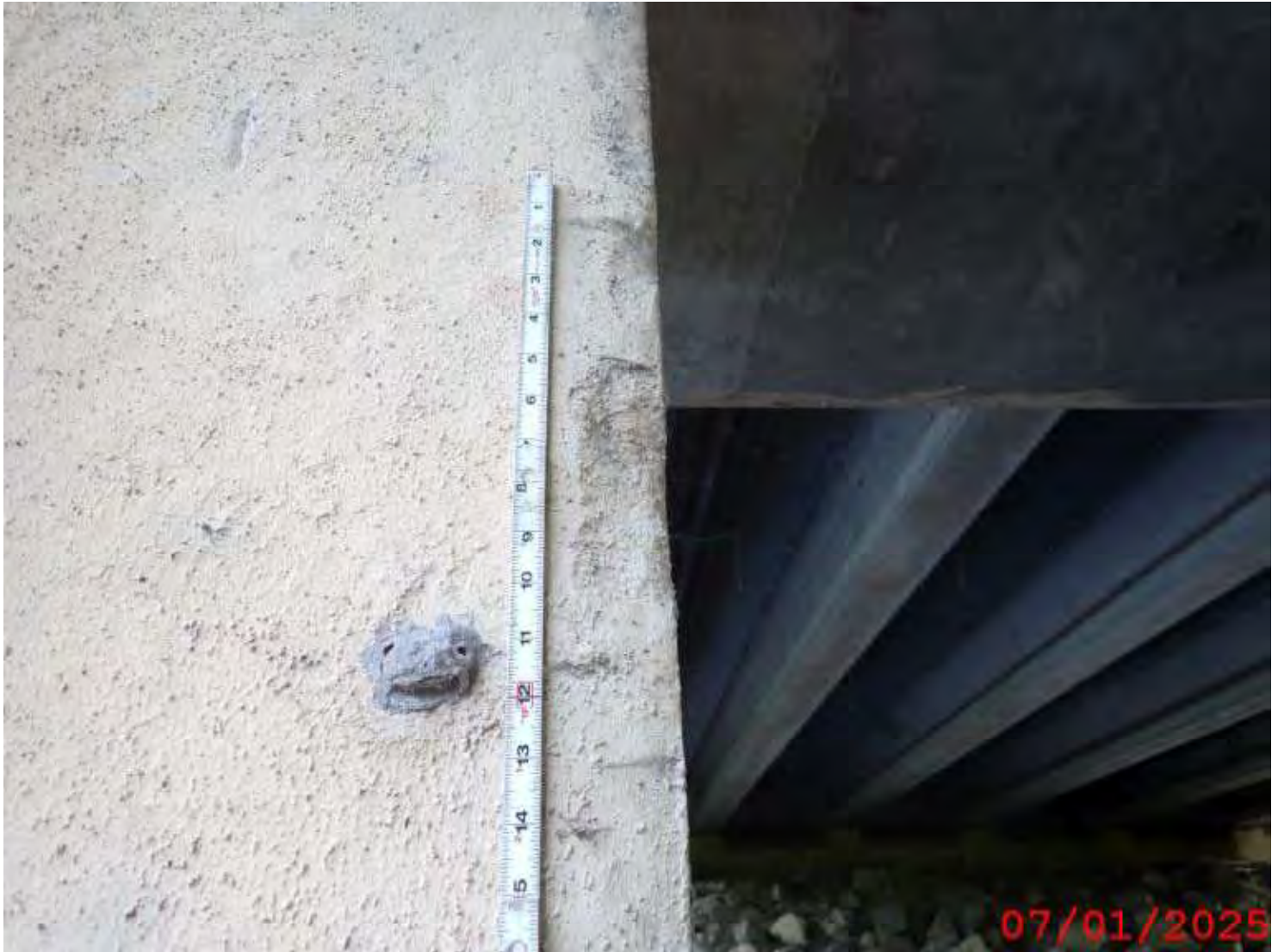
Photo 3: Element 226 Pre Conc Pile
