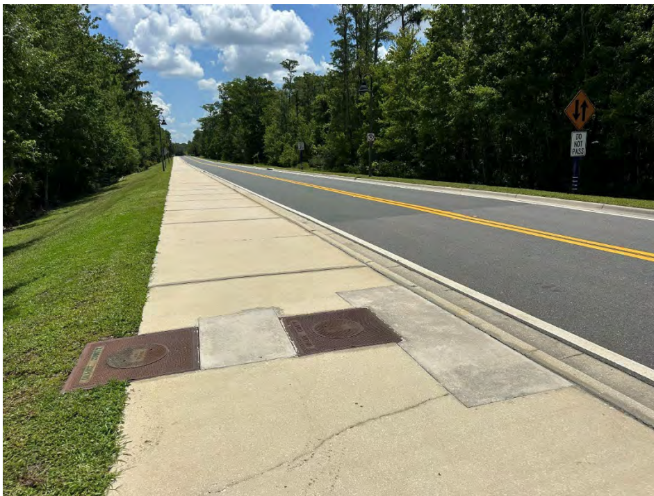
PHOTO 56 Sidewalk- broken/cracking
