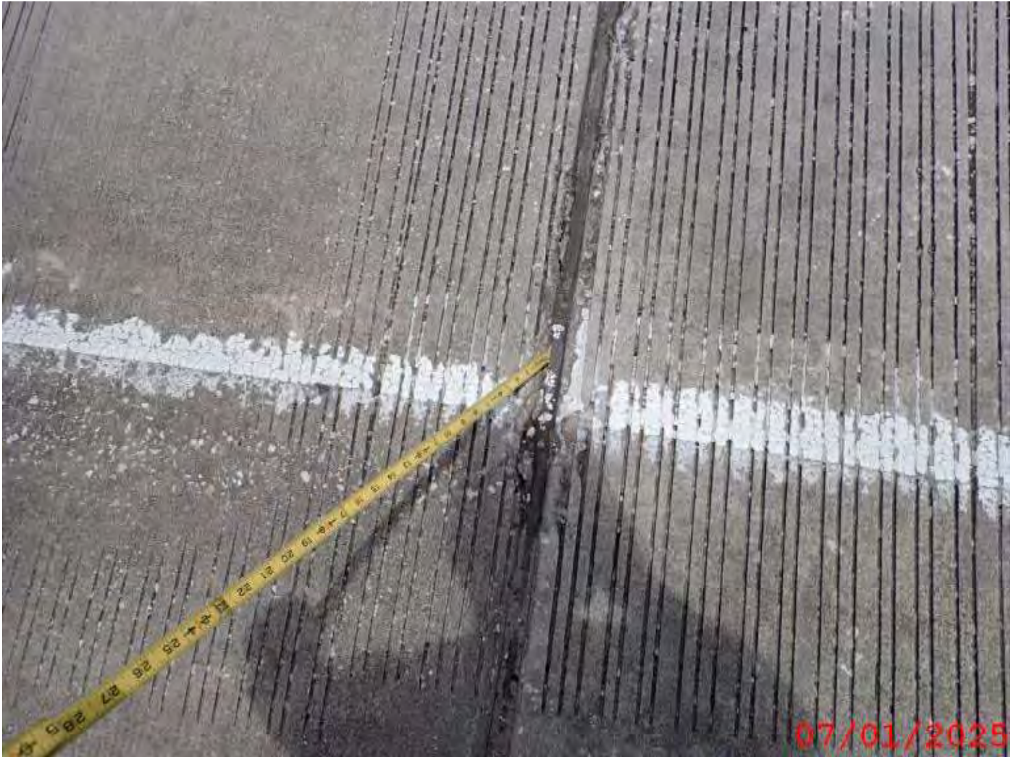
Photo 1: Element 301 Pourable Joint Seal
