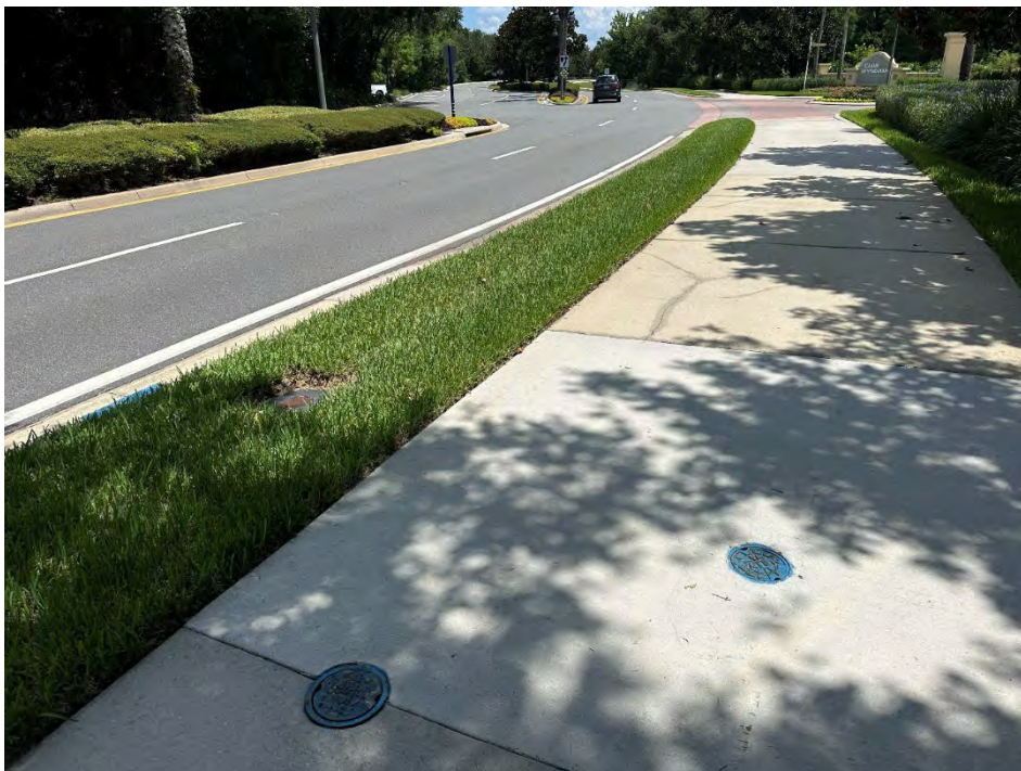
PHOTO 38 Sidewalk- broken/cracking
